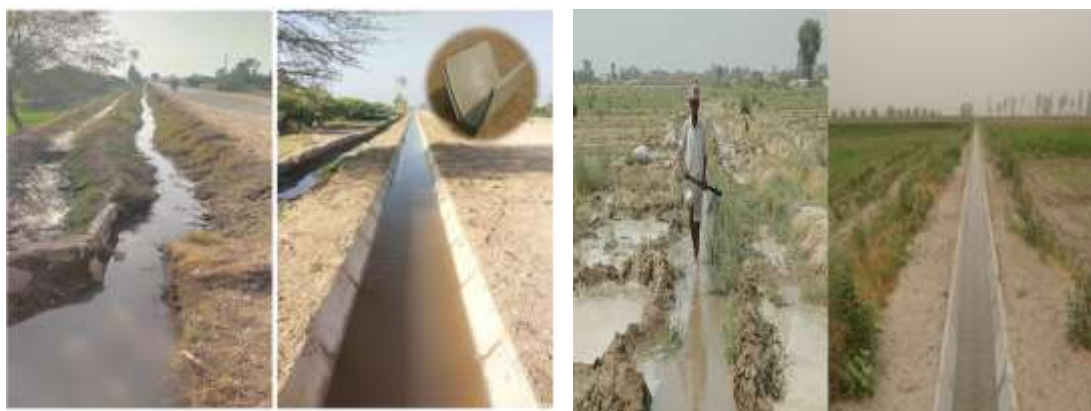
Figure 3. Glimpses of watercourses before and after lining/ improvement with PCPS technology in Punjab, Pakistan.
